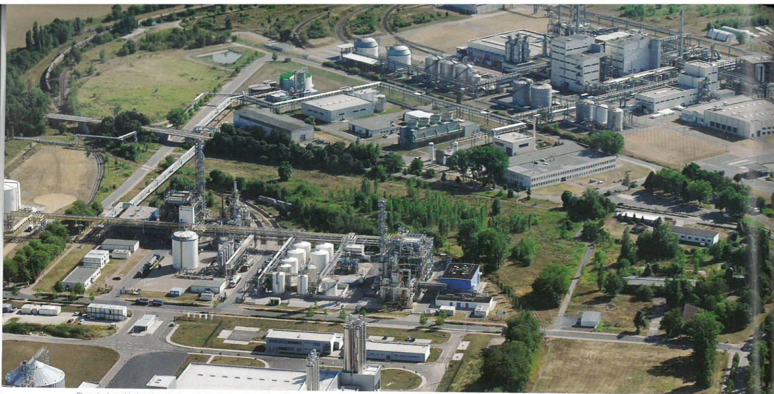
Chemical world: the chemical and industrial park in Zeitz, 40 kilometres from Leipzig
